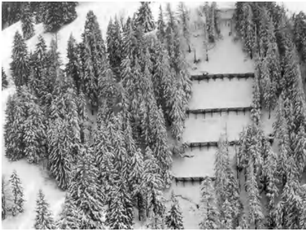
Figure 8 Avalanche starting zone in a gap within the forest protected with wooden defense structures in the Taminatal, Switzerland. The design life of such temporary wooden constructions is at least 50 years and allows time for young trees to become well established.
