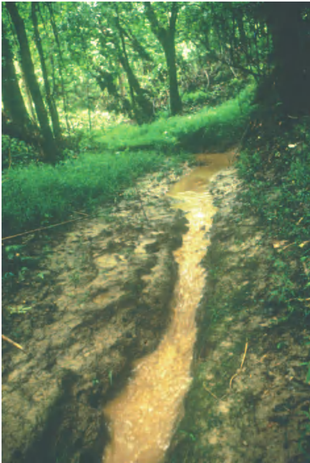
Figure 4 Improperly designed logging roads are often the source of increased levels of suspended sediment in streams.
