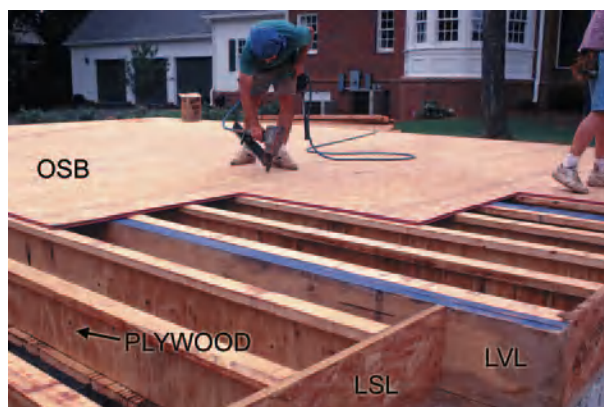
Figure 2 Structural wood-based composites used in building construction; OSB floor sheathing, LSL rimboard, I-beams with LVL as flange stock and plywood webs, and LVL floor girder. Photograph courtesy of APA – Engineered Wood Association.
