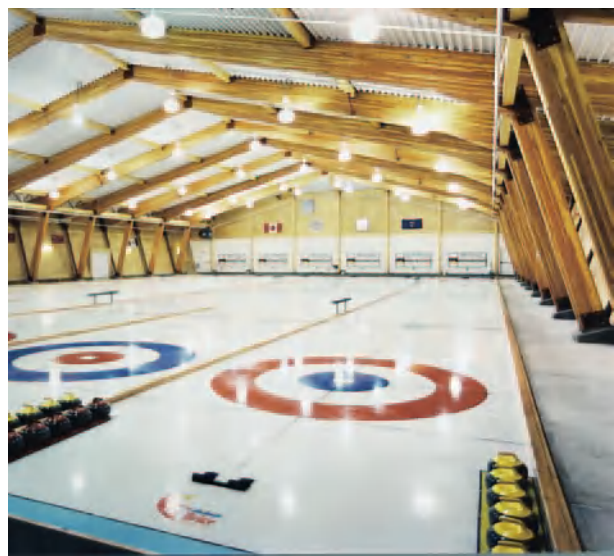
Figure 1 Glue-laminated timbers provide both structural support and pleasing aesthetics for this curling rink. Courtesy of APA – The Engineered Wood Association.
