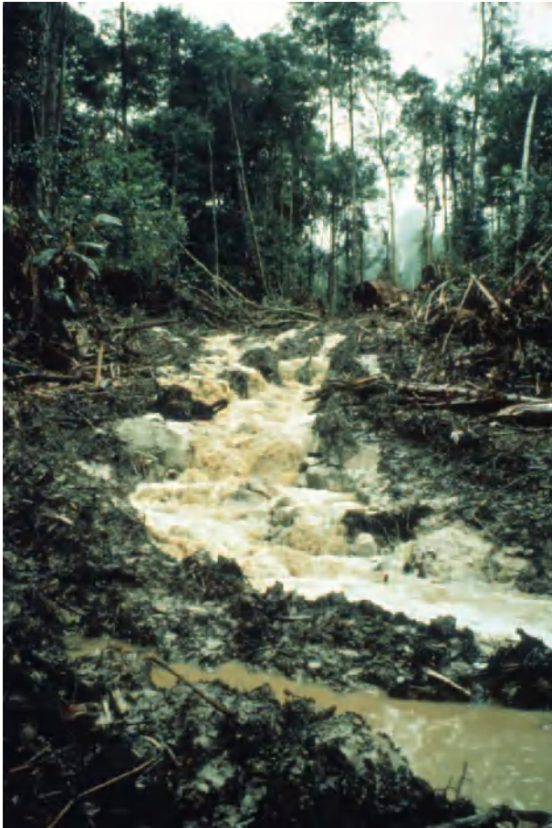
Figure 3 Overland flow develops rapidly on compacted road surfaces that have infiltration rates in some environments as low as 1 \text{ mm h}^{-1} . Photograph courtesy of A Malmer.
