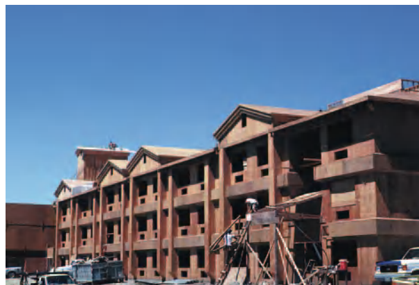
Figure 4 Plywood and oriented strand board are routinely used for roof and wall sheathing in all types of residential and commercial construction. Courtesy of APA – The Engineered Wood Association.
