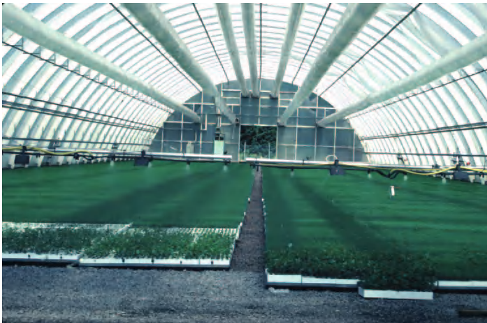
Figure 4 A single indoor unit of a container nursery in Sweden. Temperature, humidity, irrigation, and, to some extent, light can be managed in such structures. This speeds up the morphological and physiological development of the plants. Fertilization and pest control is typically done through the irrigation system, which in this case is an overhead traveling boom sprayer.
