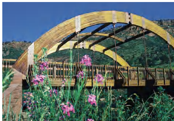
Figure 9 Hinged glue-laminated timbers support the deck of this graceful arch bridge. Courtesy of APA – The Engineered Wood Association.
